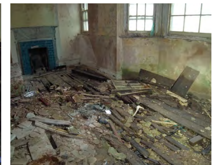
6. As with most of the building, the floors in the dormitories are unsafe and have rotted through in places. A variety of colourful fireplaces have their tiling still in place.
