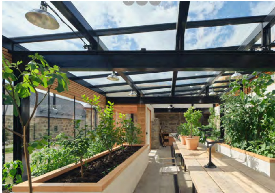
The project's glasshouse reuses an existing retaining wall (Wilson and Kennedy 2023)
