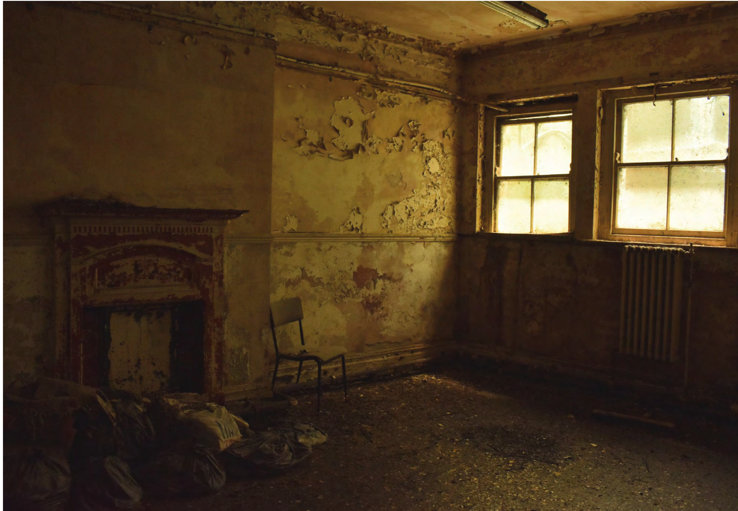
Diffused light enters the empty NUR offices (D Meurig 2021).
